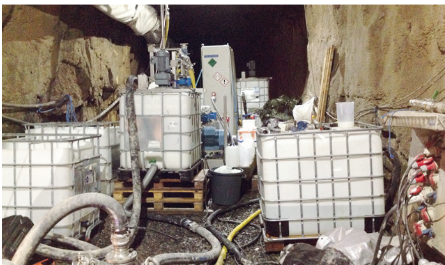
A typical setup of instruments during a sulfur removal pilot in a mine. Sulfur concentrations are analyzed in the nearby container.
